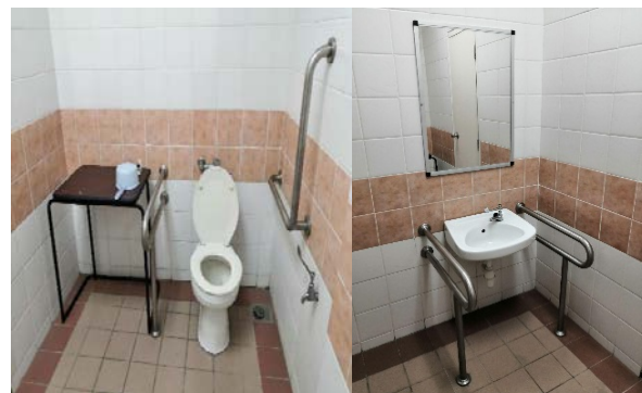
Figure 4 Toilet for a person with disabilities located at the Faculty A
