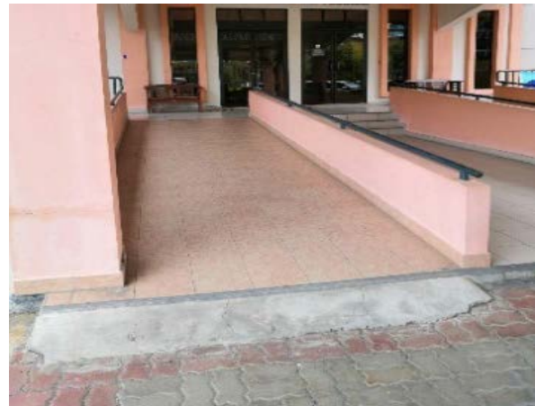
Figure 2 Ramps in the main entrance of the Faculty A
